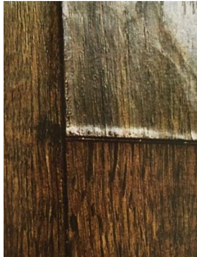
Level 4: failed test (Source: NALFA)
